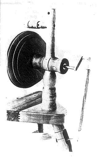
Step 2. Thread the brass crank onto the end of the main shaft. Tighten firmly and check the crank is in a "3 o'clock" position. The counterweight in the wheel will offset the weight of the treadle and permit a convenient start to spinning.
